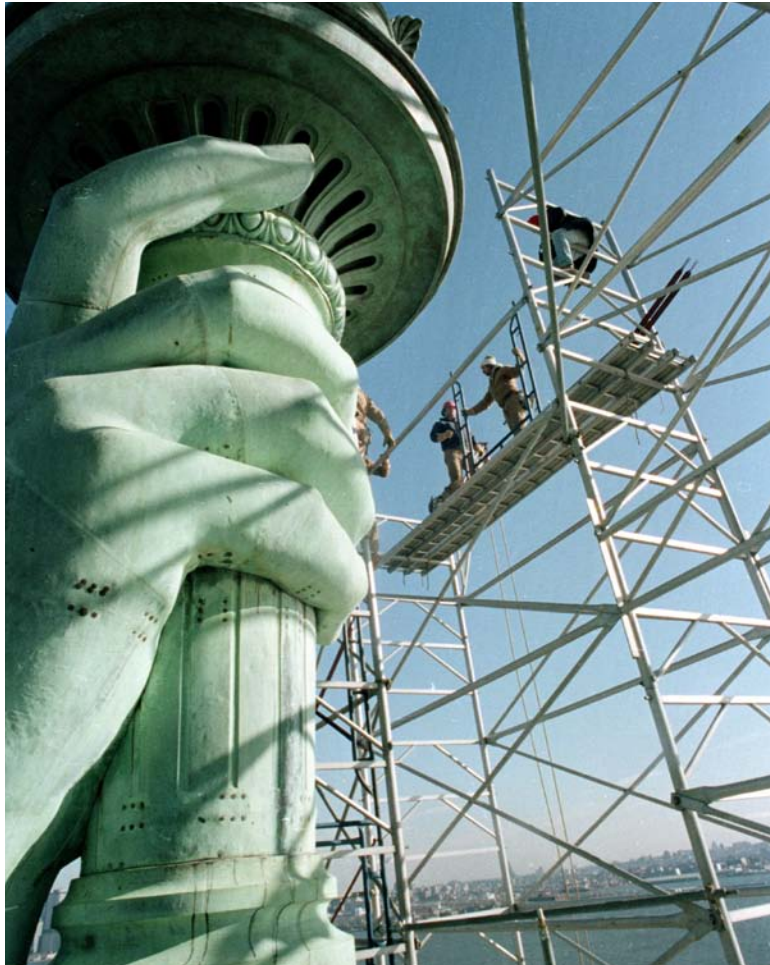
Workers fix the torch in 1985.
