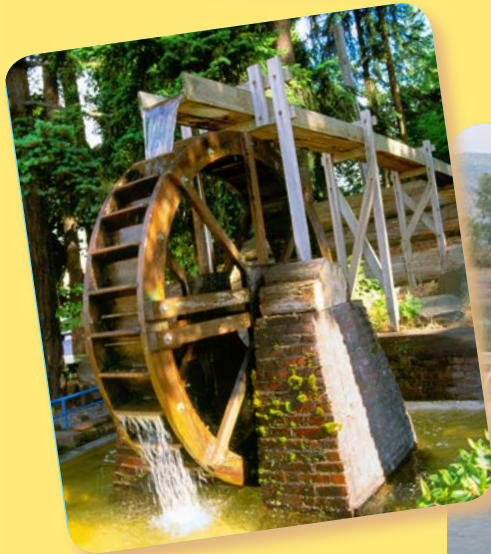
In an overshot wheel, water pushes the wheel from the top.
